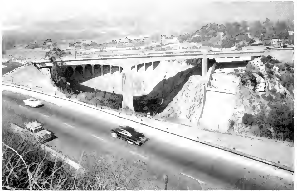
This new Devil's Gate Dam bridge eliminates old, narrow roadway as well as a sharp curve and grade intersection with Sign Route 11 at westerly end of dam
